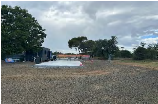
Weighbridge nears completion.
